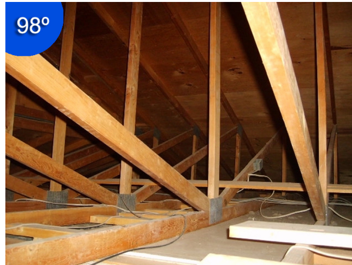
5/13/09 New roof tile over Therma Sheet. Span of IR image reduced to 91-101° F to match original 4/7/09 image. Attic temperature has been lowered 30°F with the addition of Therma Sheet.
