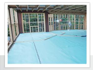
Creates a thermal break between the slab and ground, allowing slab to maintain desired temperature.
