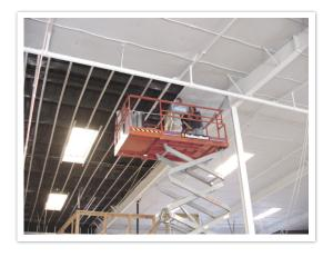
White aluminum facing provides a **clean and bright interior finish** for exposed ceilings and walls.
