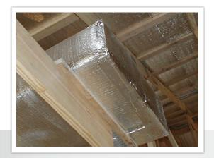
Flexible and durable duct insulation that does not absorb moisture and maintains performance values.
